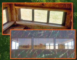
The PW Slider is a horizontal mounted operating window with three sashes. The middle sash is fixed and, the outside sashes slide towards the center. This window can be mounted from the inside or the outside.
